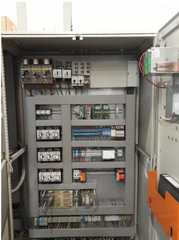
Figure 17: The switch cabinet of pump station Denglerquelle
