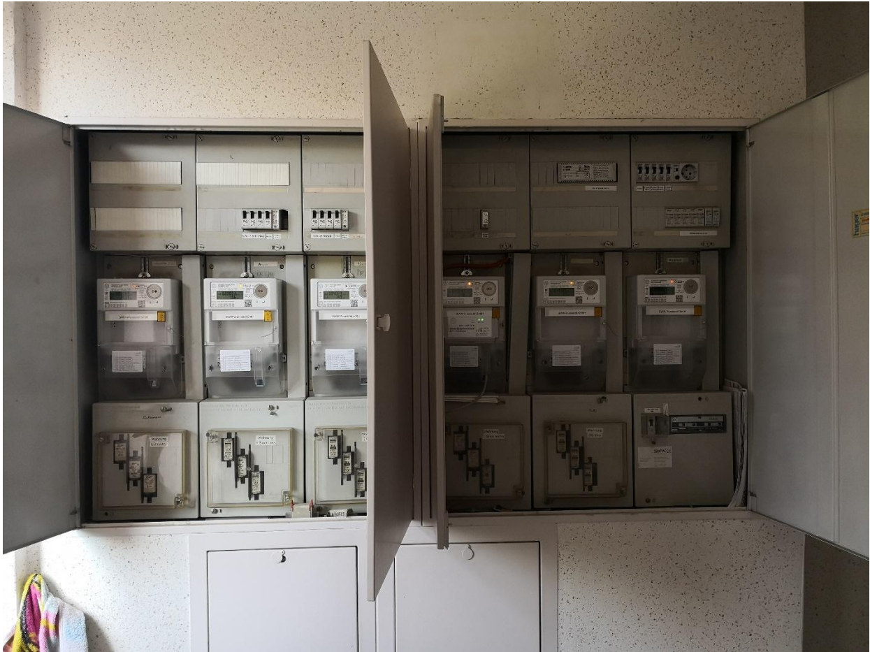
Figure 22: Picture of Controller Cabinet WunWohnlabor for ripple controller
